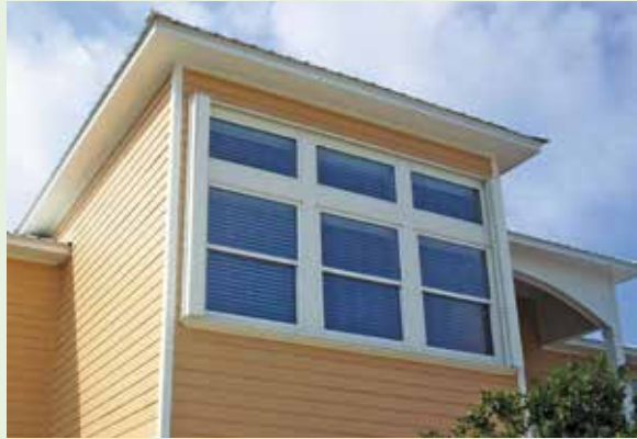
Figure 5-12. Accordion shutter (shown in the open position) installed over a large window of a coastal home. Shutter has been installed to allow deployment from inside the home. Image courtesy of Roll-a-way
