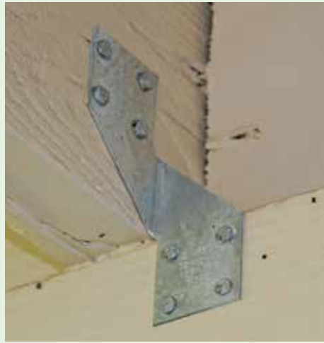
Figure 5-9. This is an example of retrofitting an existing house originally built without hurricane clips. The popular H3 clip is used here; four nails attach the clip to the roof (truss-rafter) and four more nails attach to the wall or top plate below. For a retrofit, the clips are exposed on the outside of the house; therefore, both the clip and fasteners should be corrosion-resistant and painted to blend with the exterior of the house. With the correct clip and nails, you could perform the work or, if you prefer, hire a licensed contractor. Image courtesy of Dennis Hwang
