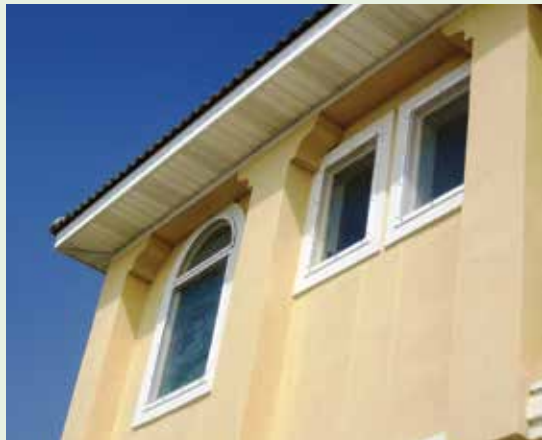
Figure 5-16. Flat impact polycarbonate panels are installed directly over windows of a coastal home. This window covering provides excellent storm protection with minimal aesthetic impact. Image courtesy of Roll-a-way
