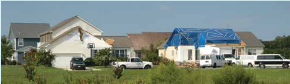
Figures 2-9. In September 2012, an EF-0 tornado with estimated maximum wind speeds of 85 mph caused structural damage in Kent County, Del. Image courtesy of Kent County Office of Emergency Management
