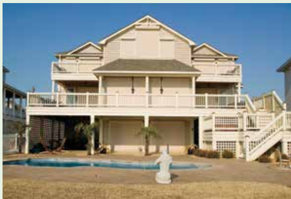
Figure 5-11. Coastal home protected with roll-down shutters on all windows and doors. The shutter is held in place by vertical guide tracks and can be deployed manually or with an integrated electric motor. Image courtesy of QMI Inc.
