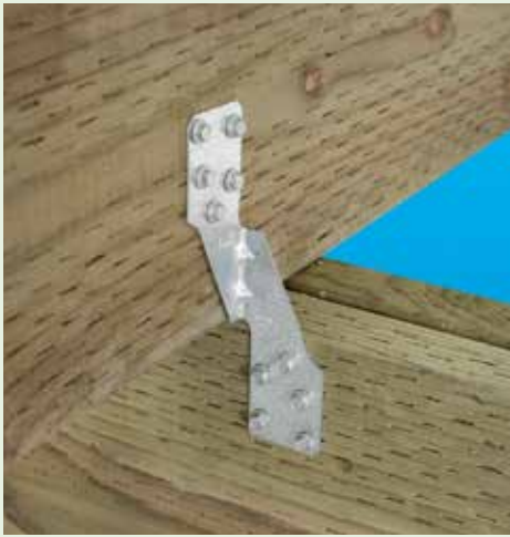
Figure 5-8. This is the popular H2.5A hurricane clip installed during new construction of houses. Five screws are driven into the lower beam (or top plate) and five more are used for the roof (truss-rafter) connection. A hurricane clip is required for each truss-rafter. Upon completion of this structure, the hurricane clip will be hidden from view. For a dollar or less in material cost, clips can be installed for both new and retrofit applications. Image © 2012 Simpson Strong-Tie Company Inc.
