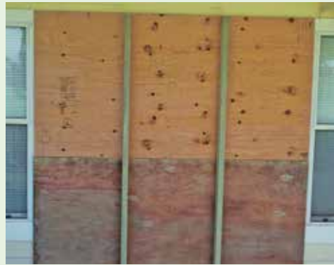
Figures 5-20 and 5-21. Not only is it necessary to install plywood opening covers correctly, it is also important to correctly label them and store them away from heat and humidity. Images courtesy of Dennis Hwang
