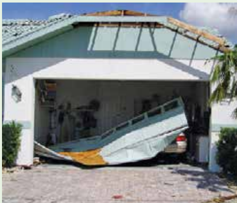
Figure 5-22. Because of their width, double-wide garage doors are more susceptible to wind damage than single doors. The wind can force it out of the roller track, especially if the track is lightweight or some of the anchor bolts are not in place. This occurs because the door fails under excessive wind pressure. You should reinforce your garage door by installing horizontal and/or vertical bracing onto each panel, using wood or light gauge metal girds bolted to the door mullions. You may also need heavier hinges and stronger end and vertical supports for your door. 4,12 Image courtesy of Florida Hurricane Depot
