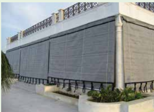
Figure 5-18. Polyethylene basket weave fabric windscreen is deployed at edge of patio, enclosing the entire area. Image courtesy of Roll-a-way
