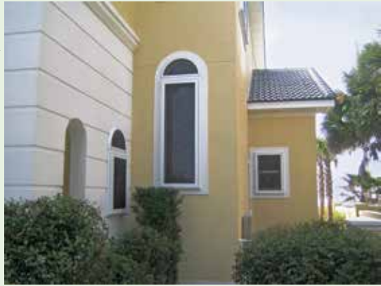
Figure 5-15. In-place stainless steel impact screen protects several windows of a coastal residence. This system requires no deployment and provides shade. Image courtesy of Roll-a-way
